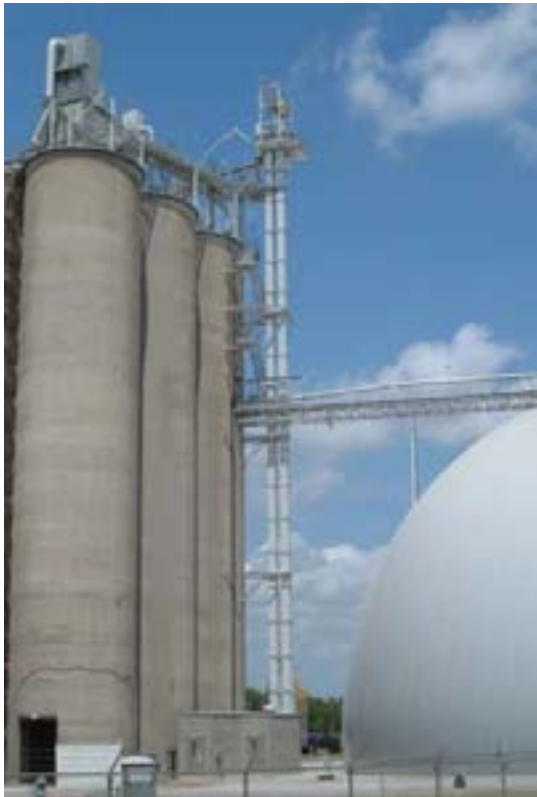
Steel cord bucket elevator: 63.5 m (208 ft - 3 in) centers
